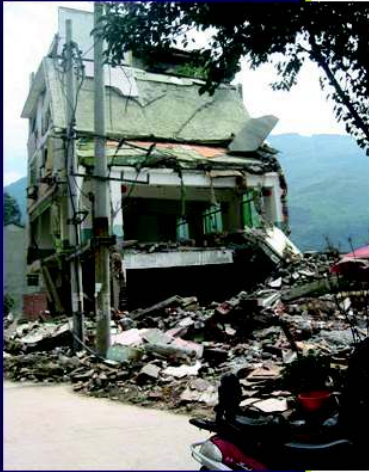
Many houses were destroyed from the 5.12 earthquake
